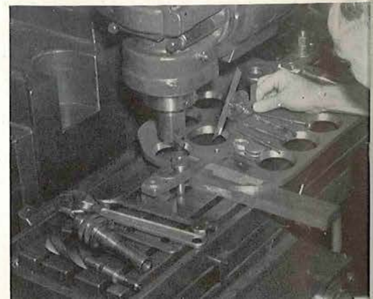
Bottom—The Van Norman demonstrates its versatility on a forming die for instrument panels.
